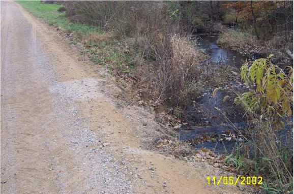
Figure 13. Crossing erosion entering Four County Drain.
